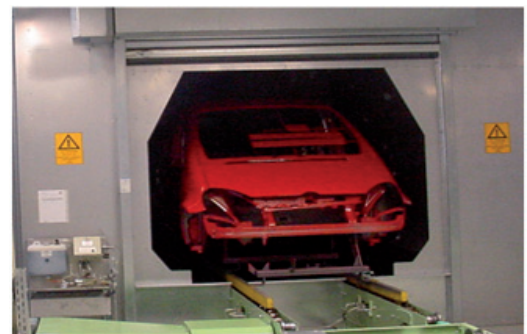
Paint shop – oven
